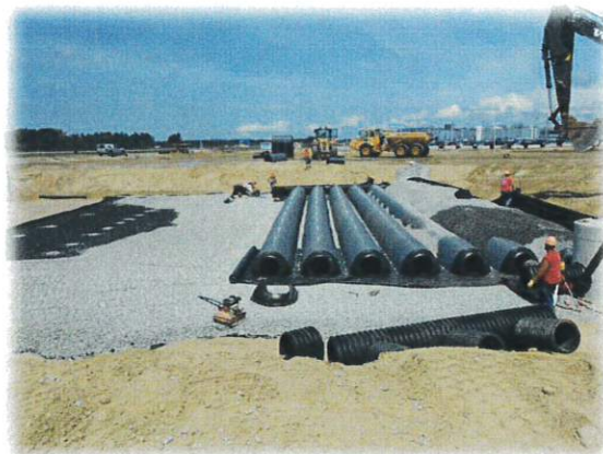
Example of Proposed Stormwater Infiltration Treatment System
