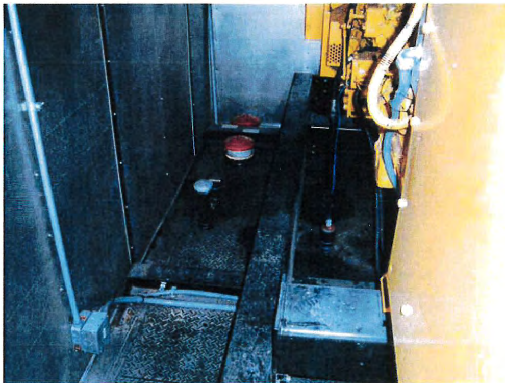
Photo #8 – Parking Garage Emergency Generator Tanks & Fill Pipe
