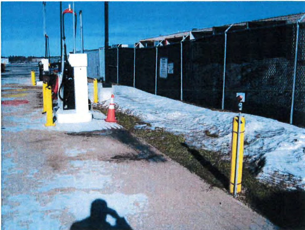
Photograph #14 – Maintenance Complex Fueling Station Emergency Shut-off
