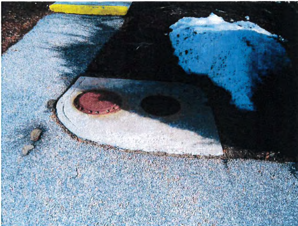
Photograph #10 – Ammon Center UST Access
