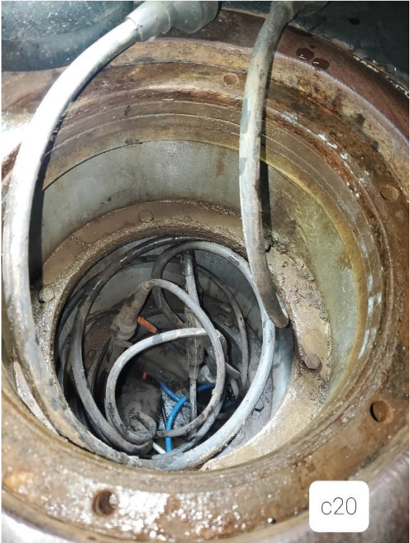
Centerline Light Fixture Base
