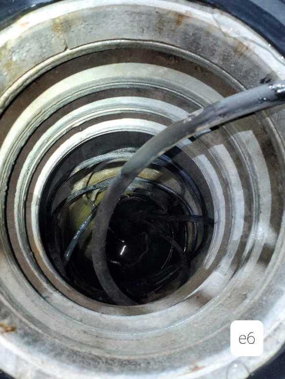
In-Pavement Edge Light Fixture Base
