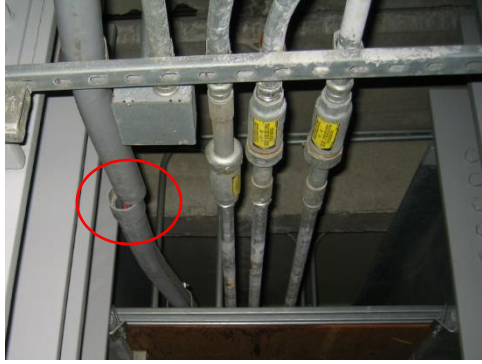
2-14 PVC conduit joint pulled apart
