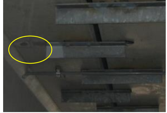
2-21 Expansion joint note where angle was cut to allow for old solar panel anchor
