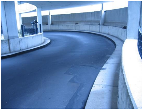
2-56 Repair in traffic coating 3 rd level
