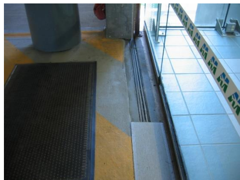
2-35 Expansion joint cover plate removed stair
