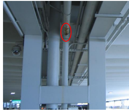
2-49 Cracked drain line at 10 th column
