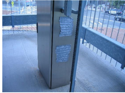
2-43 Opening in side of equipment covered with duct tape
