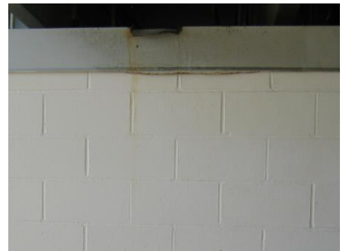
2-29 Rusted scupper southern electrical room east side.
