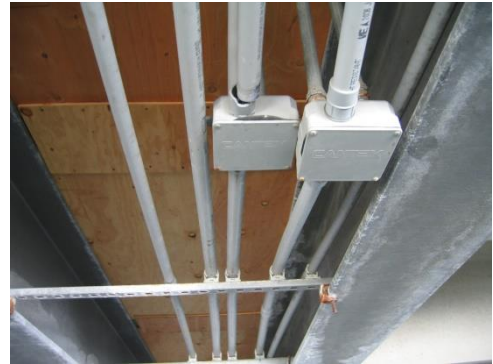
2-23 Damaged PVC electrical box and disconnected conduit
