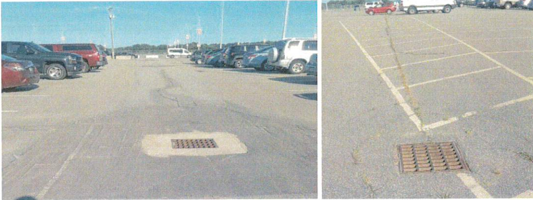
Longitudinal Cracking from Existing Catch Basins
