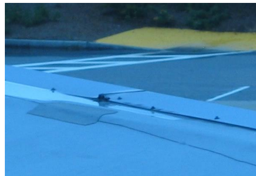
2A-3 End joint in roof edge flashing
