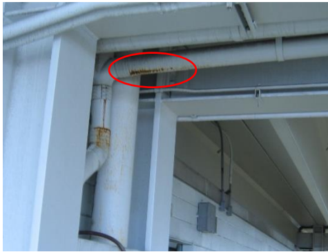
2-48 Cracked drain line
