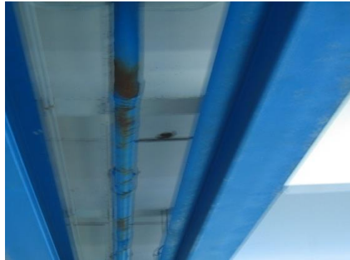
2-45 Corrosion on drain line
