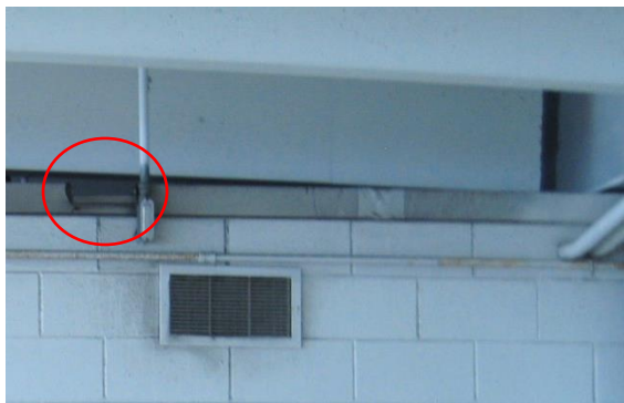
2-46 South side of National Garage office note electrical line at roof scupper
