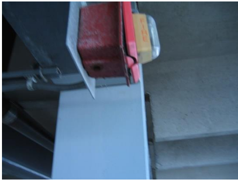
2-38 Damaged fire alarm strobe
