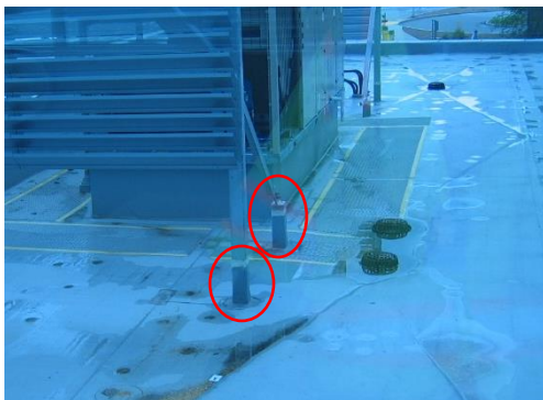
2A-2 Air handler screen support flashing
