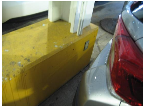
2-55 GFCI outlet missing weather cover
