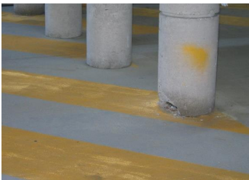
2-34 Damage concrete bollard typical
