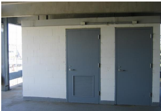
2-28 Louver in electrical room door
