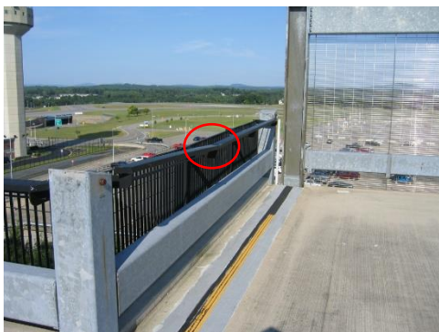
2-4 Dents in top rail west side of garage
