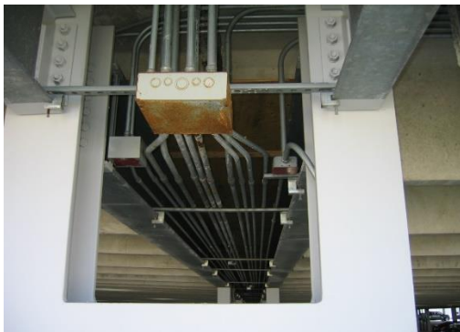
2-16 Electrical junction box rusted cover
