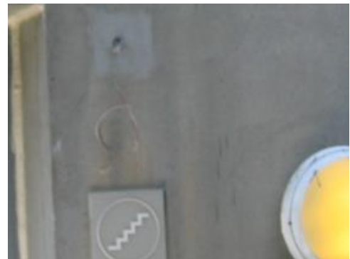
2-13 Wires from fire alarm strobe hanging out of wall.
