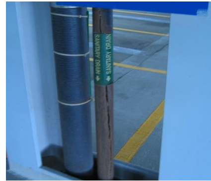
2-39 Split vertical drain pipe
