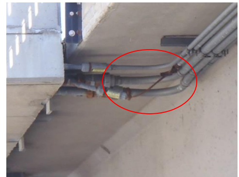
2-17 Conduit rusted through exposing wire
