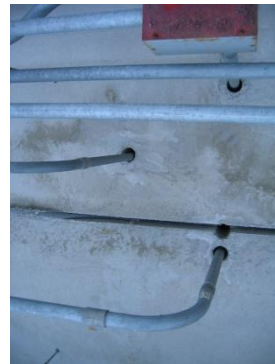
2-37 Close up of openings without fire stop
