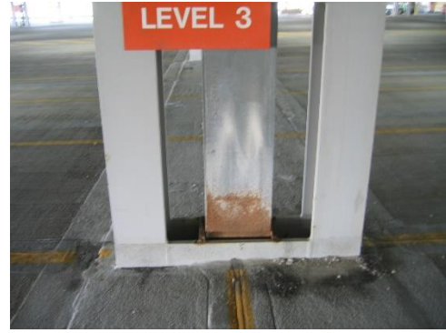
2-31 Rusted ductwork at floor level
