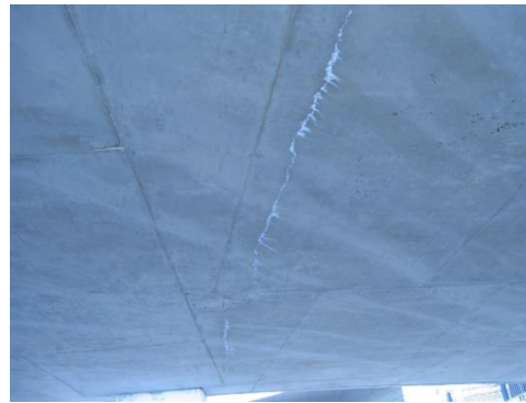
2-57 Crack with efflorescent in ceiling of helix
