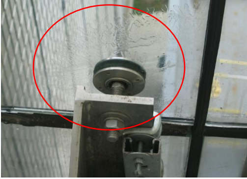
2-58 Apparent delaminating of glass wall north side of 6 th level elevator lobby
