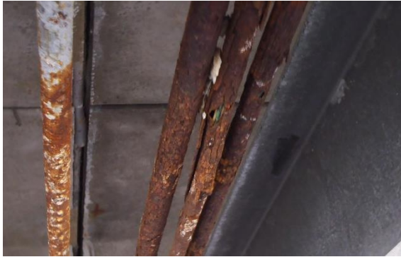
2-32 Conduit rusted through
