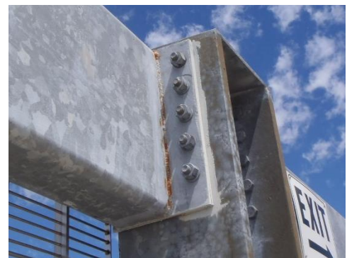
2-5 Typical rust on welded connection
