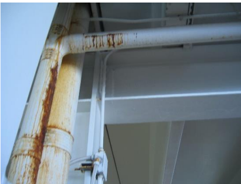
2-50 Crack in drain line
