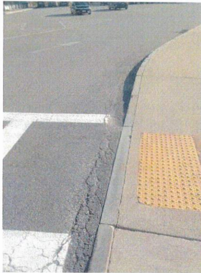
Alligator cracking along curb
