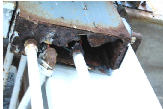
2-51 Deteriorated electrical junction box
