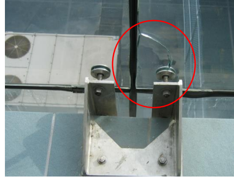
2-59 Crack in glass wall panel south side of 6 th level elevator lobby
