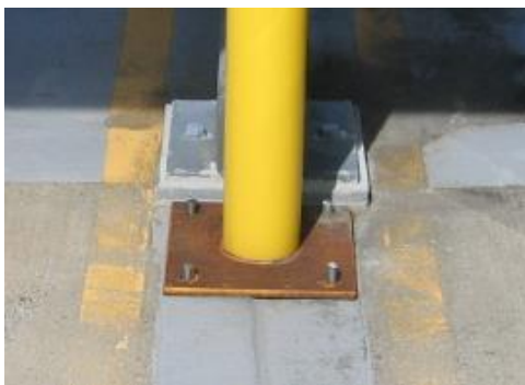
2-6 Solar panel base plate startling precast seam
