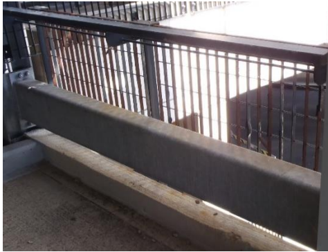
2-22 Rusted metal screen at 4 th level southern end west side of helix
