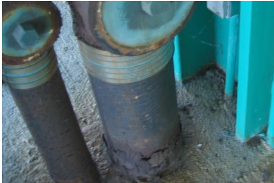
2-44 Corrosion at base of drain pipe
