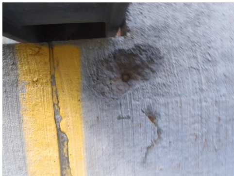
2-12 Spall in precast deck
