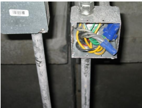
2-24 Open electrical box with exposed wires
