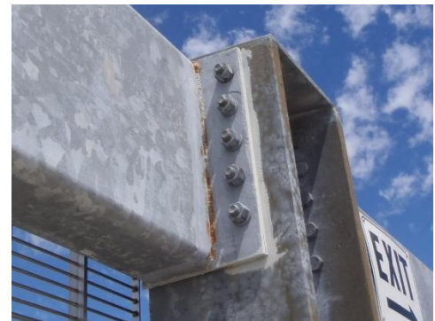
2-5 Typical rust on welded connection
