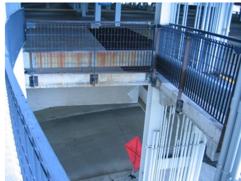
2-41 Rusted metal screen at 2 nd level southern end east side of helix
