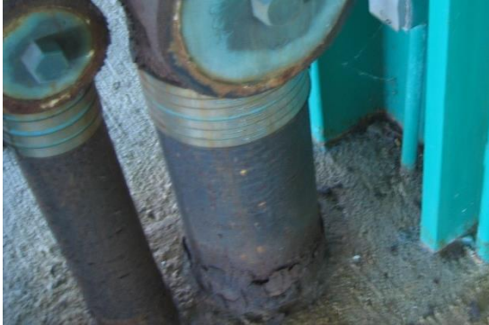
2-44 Corrosion at base of drain pipe
