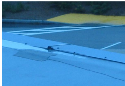
2A-3 End joint in roof edge flashing
