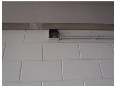
2-47 Open electrical box on south side of National Garage office
