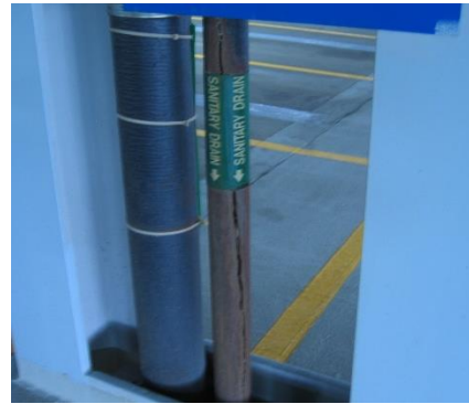
2-39 Split vertical drain pipe
