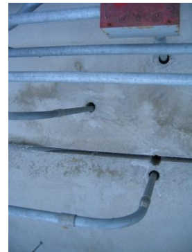
2-37 Close up of openings without fire stop
