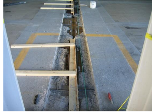
2-33 Concrete repair on C parking line
