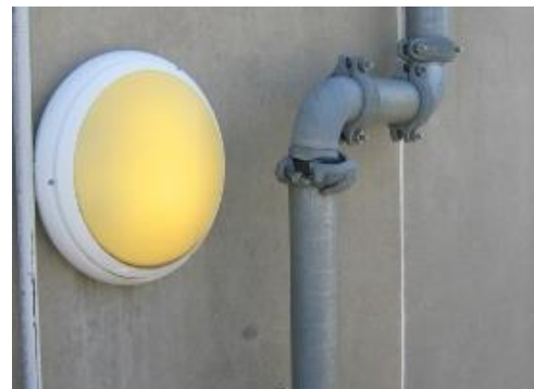
2-9 Broken conduit connection at stair 1
