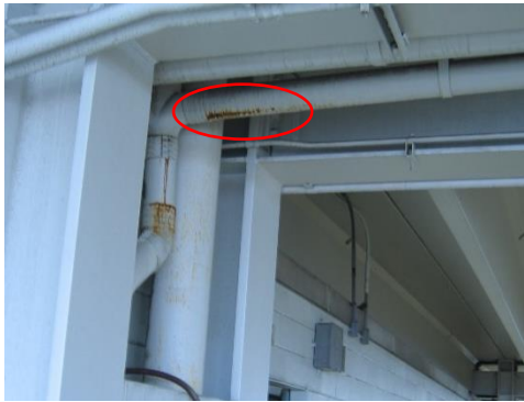
2-48 Cracked drain line
