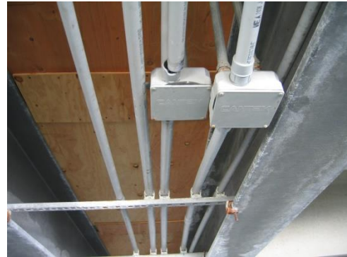
2-23 Damaged PVC electrical box and disconnected conduit
