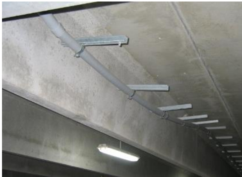
2-18 Conduit supports not fastened
