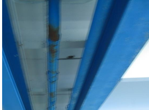
2-45 Corrosion on drain line
