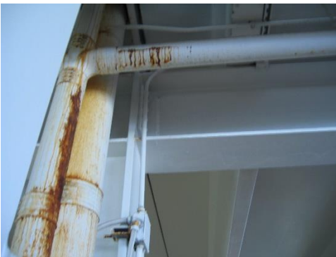
2-50 Crack in drain line
