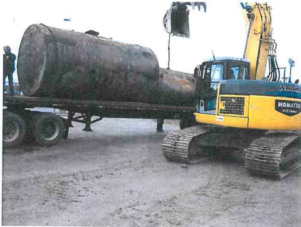
Photograph #14 – Excavated Tanks
