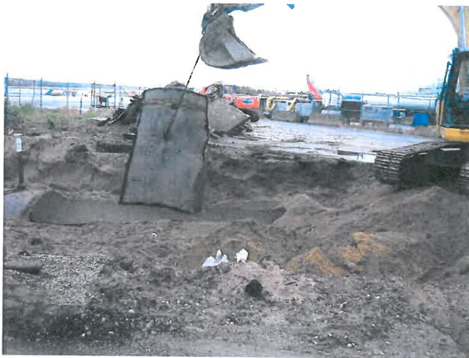
Photograph #19 – Opening 50,000-Gallon Tanks
