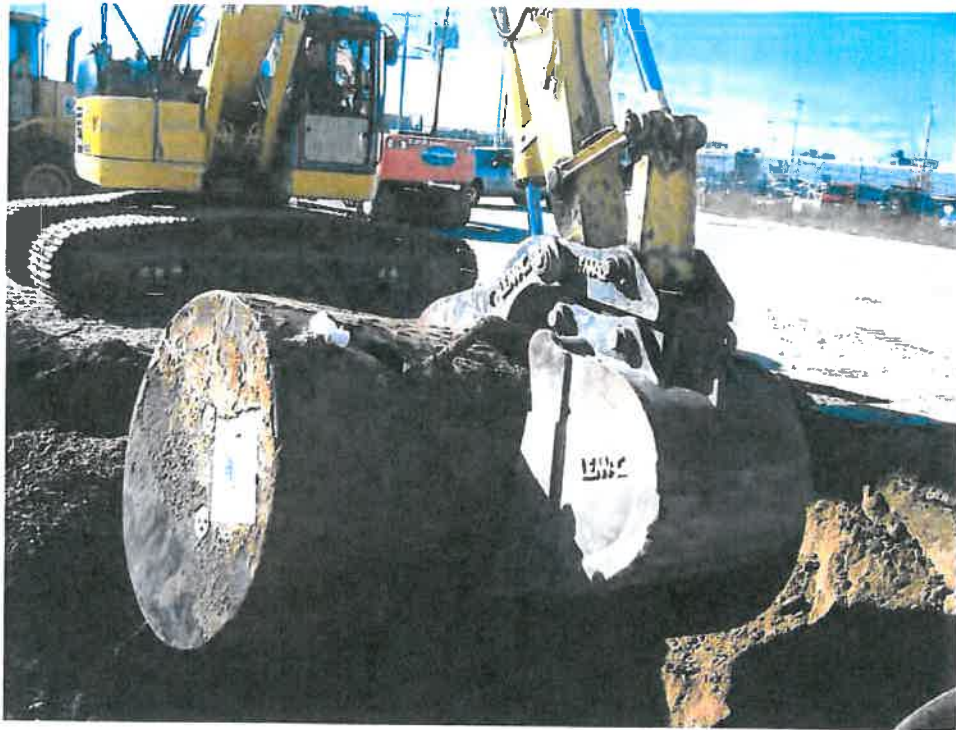
Photograph # 13 – 2,000-Gallon Tank Removal
