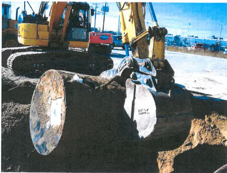
Photograph # 2 – 2,000-Gallon Tank Removal
