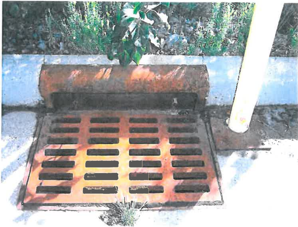
Photograph #5 – Catch Basin with Hooded Outlet
