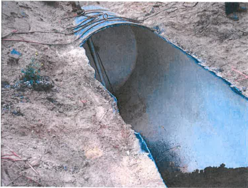
Photograph #4 – Interior of Exposed 50,000-Gallon Tank
