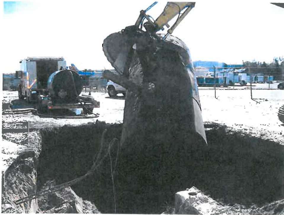
Photograph #12 – 6,000 Gallon Tank Removal
