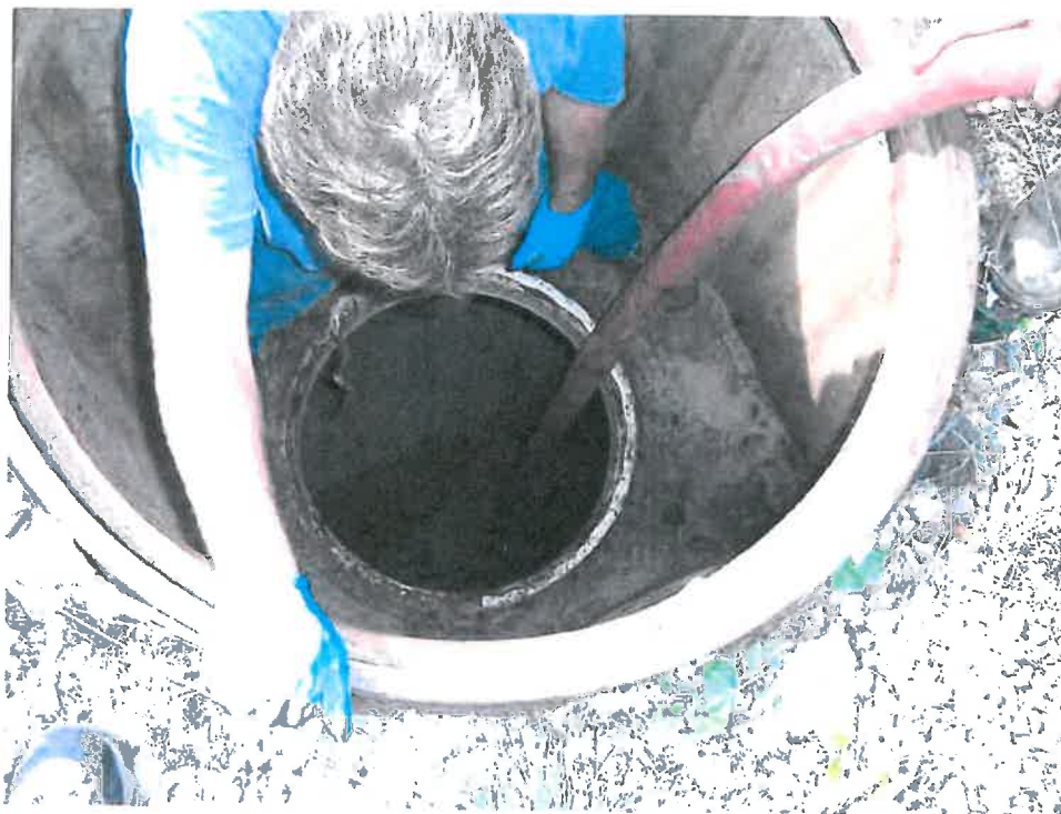
Photograph #7 - Pumping Fluid from 6,000-Gallon Tank
