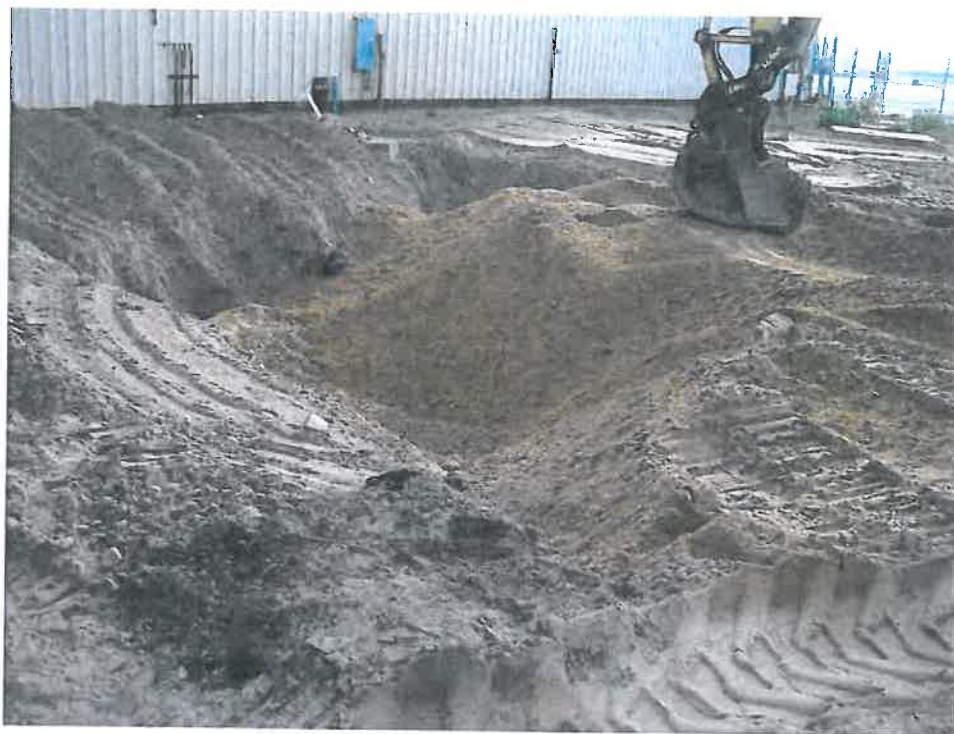
Photograph #23 – Backfilling 50,000-Gallon Tank Excavation
