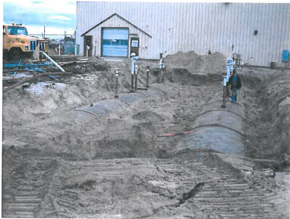
Photograph # 18 – Excavated 50,000-Gallon Tanks
