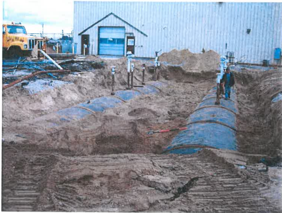
Photograph # 3 – Excavated 50,000-Gallon Tanks
