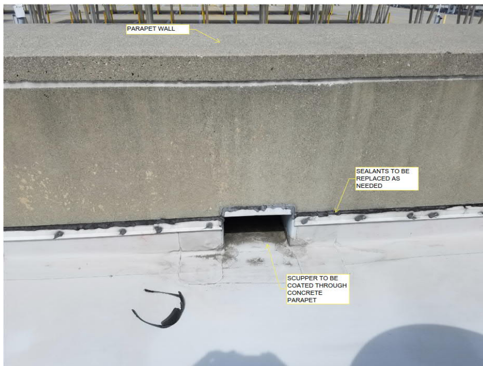
PHOTO 12 STAIR TOWER ROOF CUPPER
