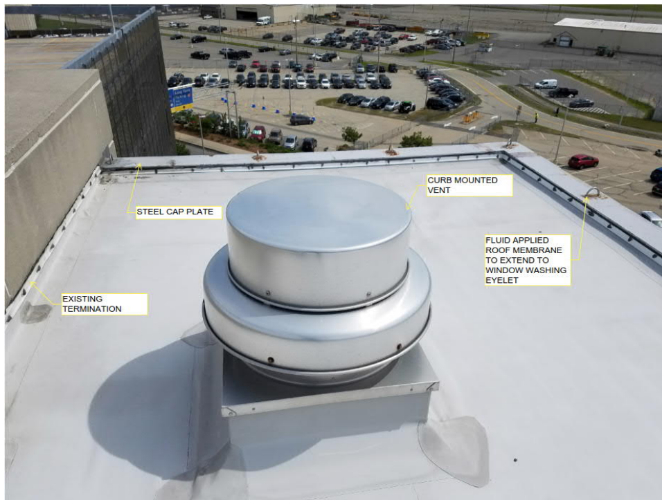
PHOTO 11 TYPICAL STAIR TOWER ROOF
