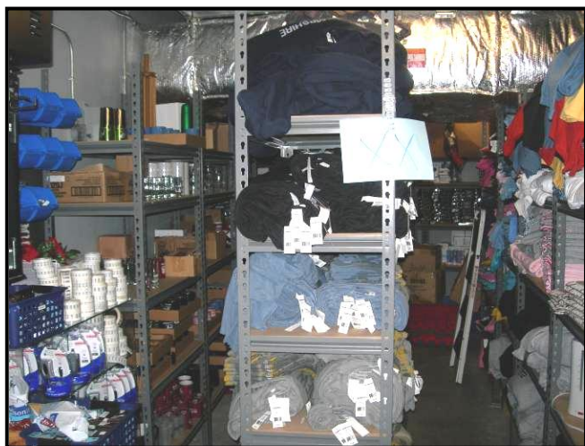
FIGURE 7.2-9 MECHANICAL ROOM USED FOR CONCESSION STORAGE
