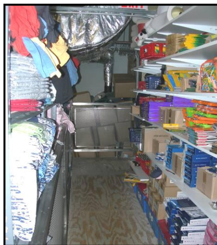
FIGURE 7.2-10 MECHANICAL ROOM USED FOR CONCESSION STORAGE
